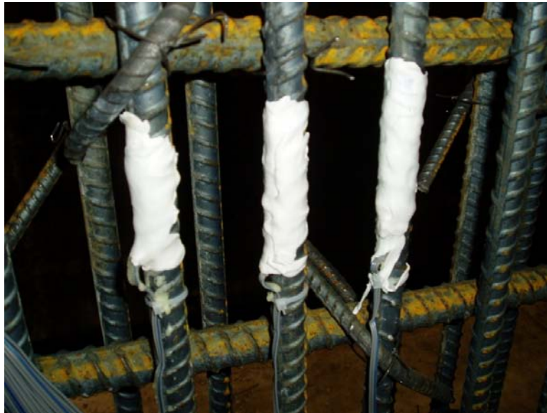
Figure 6-22: Application of the second layer of coating protection, SB tape..
