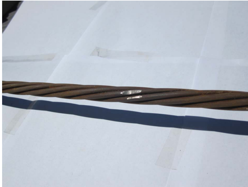
Figure 6-18: A typical seven wire 0.6-in. diameter strand after being grinded to host a strain gage.
